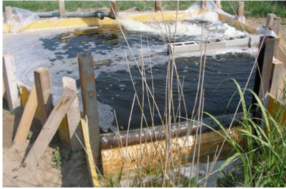
Figure 6: The upstream weir at the head tank.
