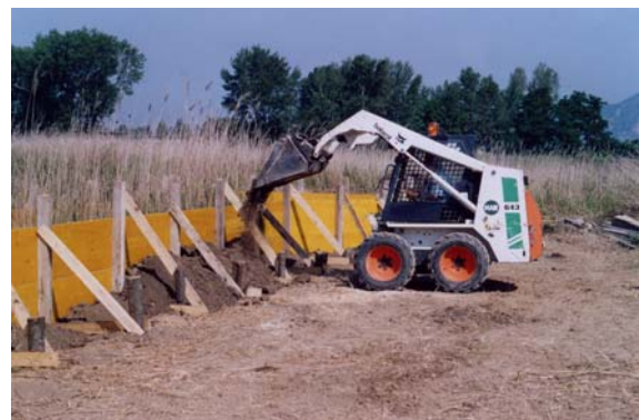
Figure 5: Construction of the lateral levees.
